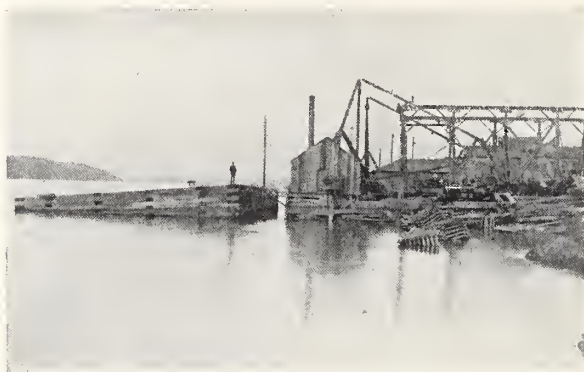
Bridge Caisson, Ready to float to Position, 1877.
